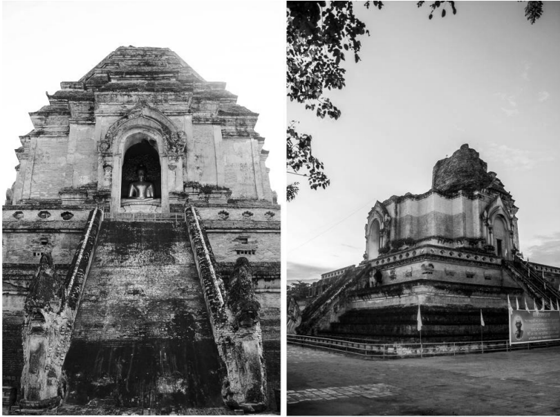
<Fig. 4> Current architectural condition of the Grand Stupa with its damaged superstructure, Wat Chedi Luang
